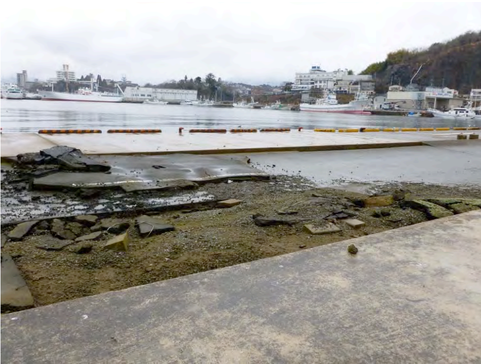
Figure 2 – Pile-supported dock with local subsidence failure of dockside infill: Kesenuma Port, Japan, March 10, 2012, one year after tsunami.
