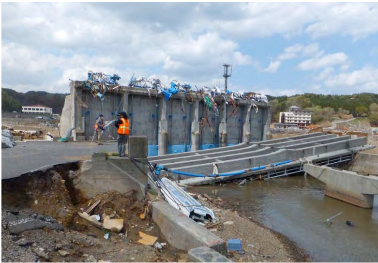
Figure V-4: Field survey of Iwate Prefecture Japan. Georeferenced Photo label is: DSCF0248_5-13-11_Taro Fishing Port_Bridge Deck System Turned Upside Down off Piers Adjacent to Canal Control Structure_RMN.JPG
